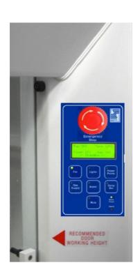
The EcoAir® III Controller comes with a vertically oriented, touch-type control panel that can be mounted on either the left or right column of a fume cupboard. This example shows the control panel mounted on an EcoAir® fume cupboard.
